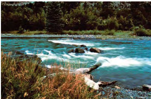
Figure 11-33 W-weir installed on the Uncompahgre River, CO
